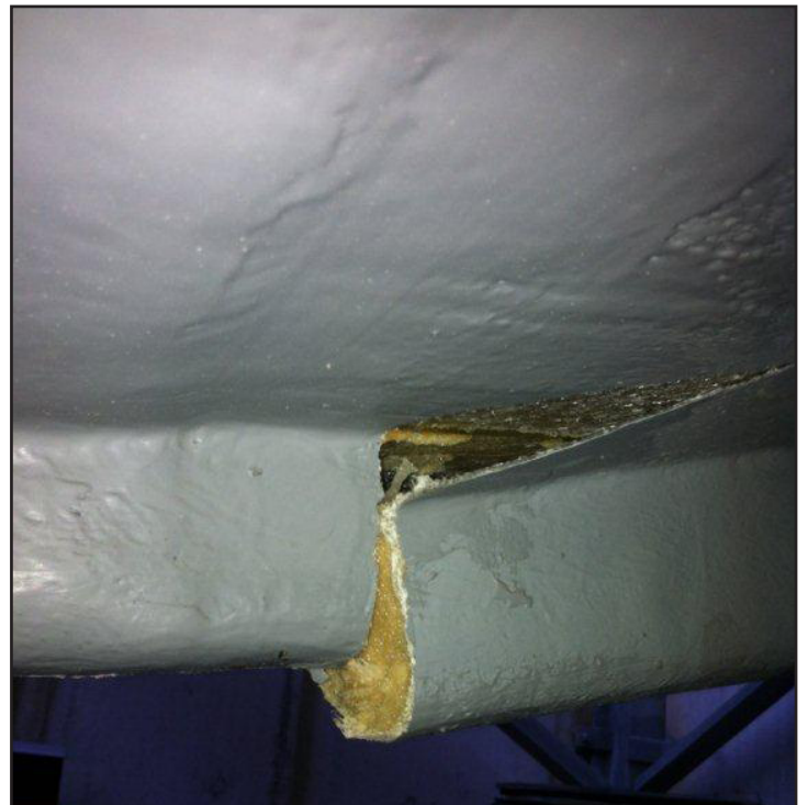
Cracked basin on RCT cooling tower.
