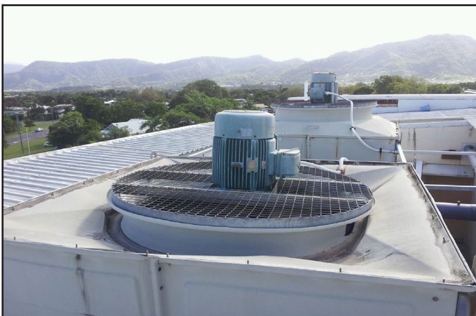
Collapsed fibreglass fan cylinder on competitors IL cooling tower.
