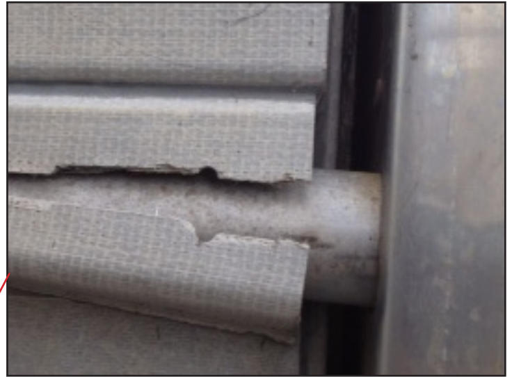
Cracked casing panel on competitors RCT cooling tower.
